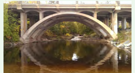
North Shore Scenic Drive bridge over the French River
